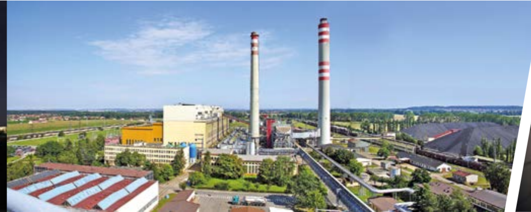
Opatovice nad Labem power station
